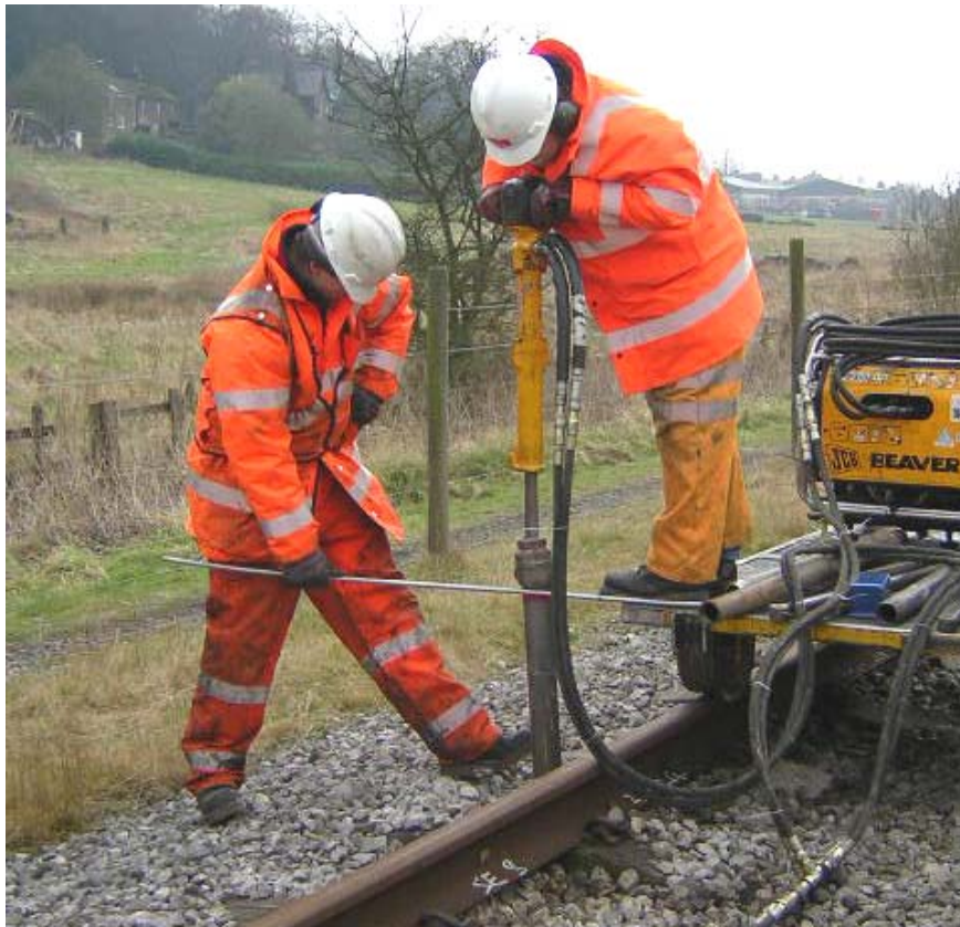
Figure 3: Intrusive trackbed investigation - Automatic Ballast Sampling (ABS).
